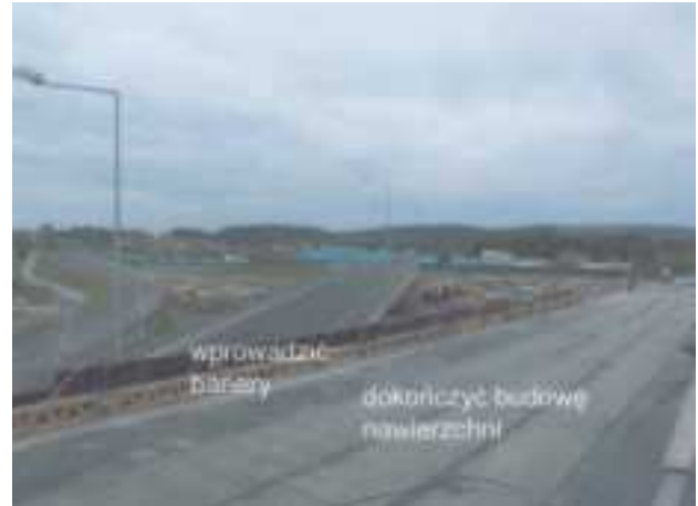
Figure 5a: The “before” view of the road construction.
