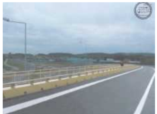
Figure 5b: The “after” view of the new road segment, in which pavement, road lanes, safety railings and barriers were designed, creating the graphical simulation of the future road picture.
