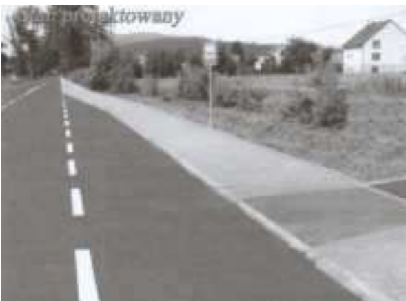
Figure 2c: The “after” view of the reconstructed road, in which new edge lines were painted, the bus stop and bus lane was created and the aesthetic pavement was designed with the junction road in the middle.
