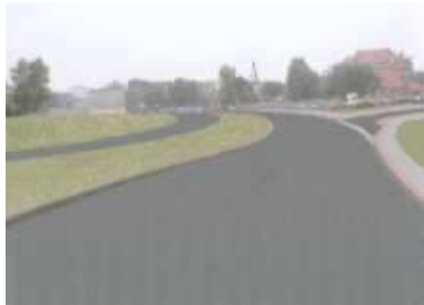
Figure 1b: The final effect “after” designing the new road segment geometry and the road architecture.
