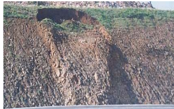
FIGURE 5 ROTATIONAL SLIDE AFFECTING A SLOPE OF BASALTIC SOIL
